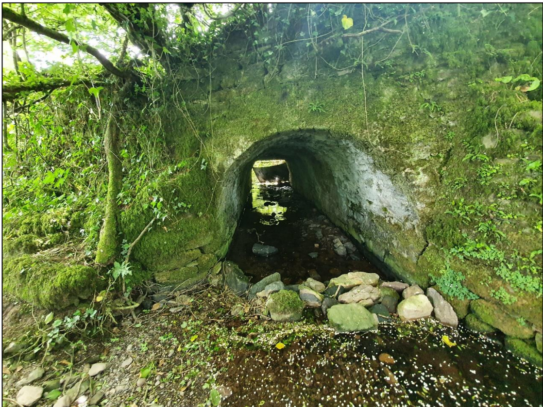
Plate 4-19 The Glennaglogh River, located along the turbine connector route, which will be located within the existing road over the bridge.
